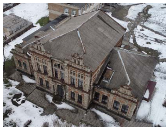
Fig. 1. Aerial overview of the building
